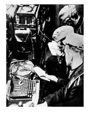
The Enigma machine looked like a typewriter in a wooden box. An electric current went from the keyboard through a set of rotors and a plugboard to light up the 'code' alphabet.
